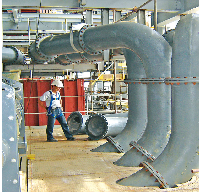
Typical applications of KALMETALL-C hard casting are pipe systems; here the pulverized-coal pipe of a power plant in South East Asia
