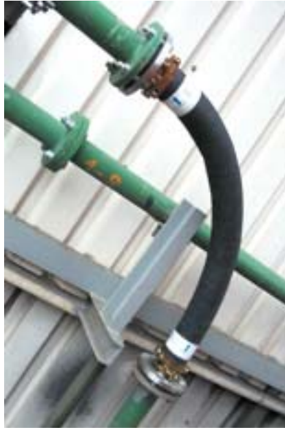
KALFLEX are flexible pipe bends with abrasion resistant segments
