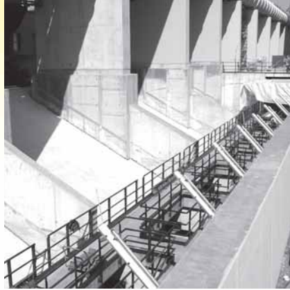
Lining of a coke-loading bay with tiles made of KALSICA-P:
