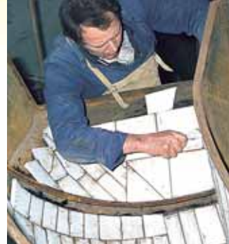
Chutes lined with KALCERAM are a solution that lasts, e.g. for bag loading systems in cement plants
