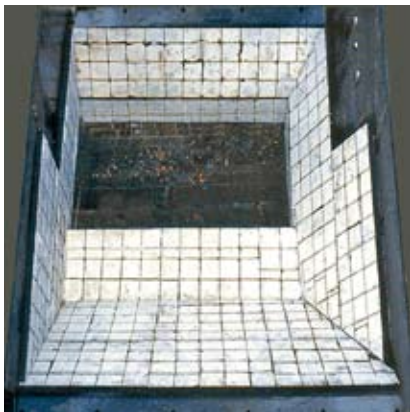
Bunker in a steel mill lined with KERAFLEX-KRM elements
