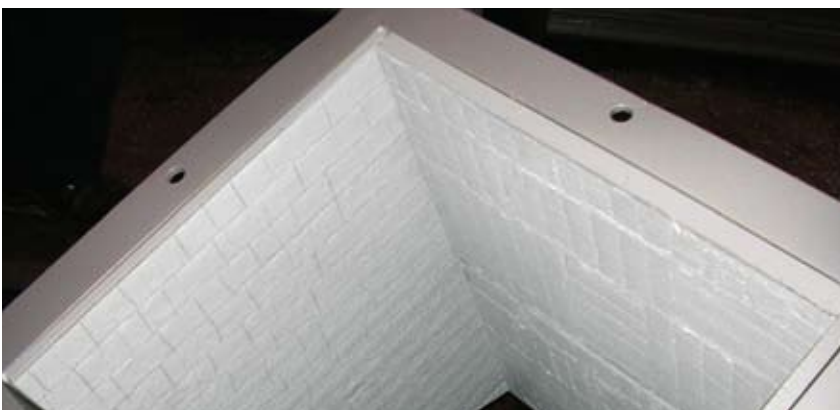
Bunker in a cement plant: the KERAFLEX-WRM elements consist of 5 mm carrier plate, 5 mm rubber and 13 mm KALMETALL-W hard-overlay welding (8 + 5)
