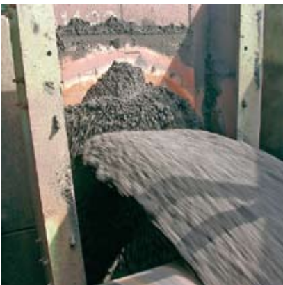
KERAFLEX-KRM installed as protection against abrasion and impact load in a discharge chute for coal and iron ore in a harbor loading and unloading plant
