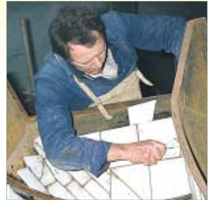
Chutes lined with KALCERAM are a solution that lasts, e.g. for bag loading systems in cement plants.
